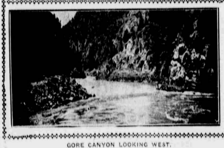
GORE CANYON LOOKING WEST.
