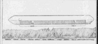
The latest invention to traverse the upper regions independently of a currents is that of Count Zeppelin, which was tosted a little while and made a voyage of 35 miles without mishap. The airship proper is 420 flors and 37 feet in diameter, with a capacity of 400,000 cubic feet. It was 7,260 pounds and is propelled by two 15 horsepower motors fixed on cars wh
