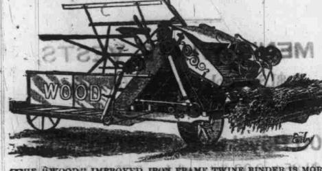
THE "WOOD" IMPROVED IRON FRAME TWINE BINDER IS MORE simple in construction, has fewer parts, and is the most perfect automatic Self Binder ever put upon the market. Upon the following points we challenge comparison: DURABILITY, SIMPLICITY, EASE OF MANAGEMENT AND ADJUSTMENT, LIGHTNESS OF DRAFT, CERTAINTY OF BINDING, SECURITY OF KNOT TIED.
