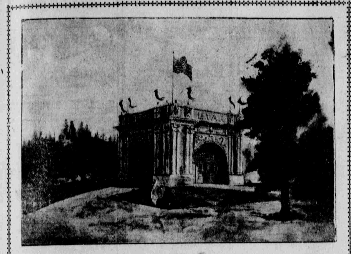
UTAH PAVILION TO BE ERECTED AT ST. LOUIS.
