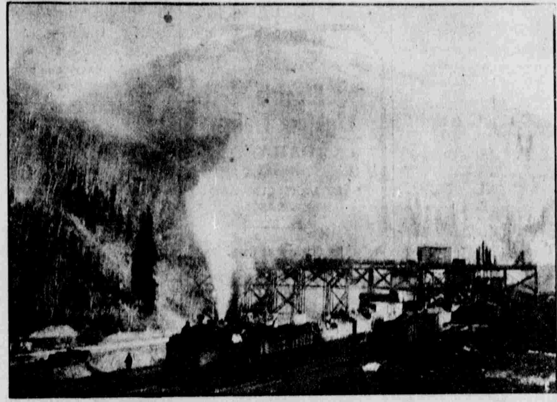
CLEAR CREEK COAL YARDS AND TIPPLE.
