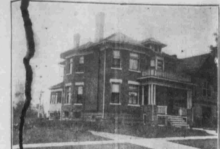
This new modern 11-room brick, near St. Mary's Cathedral, for $14,000. Terms to suit.
