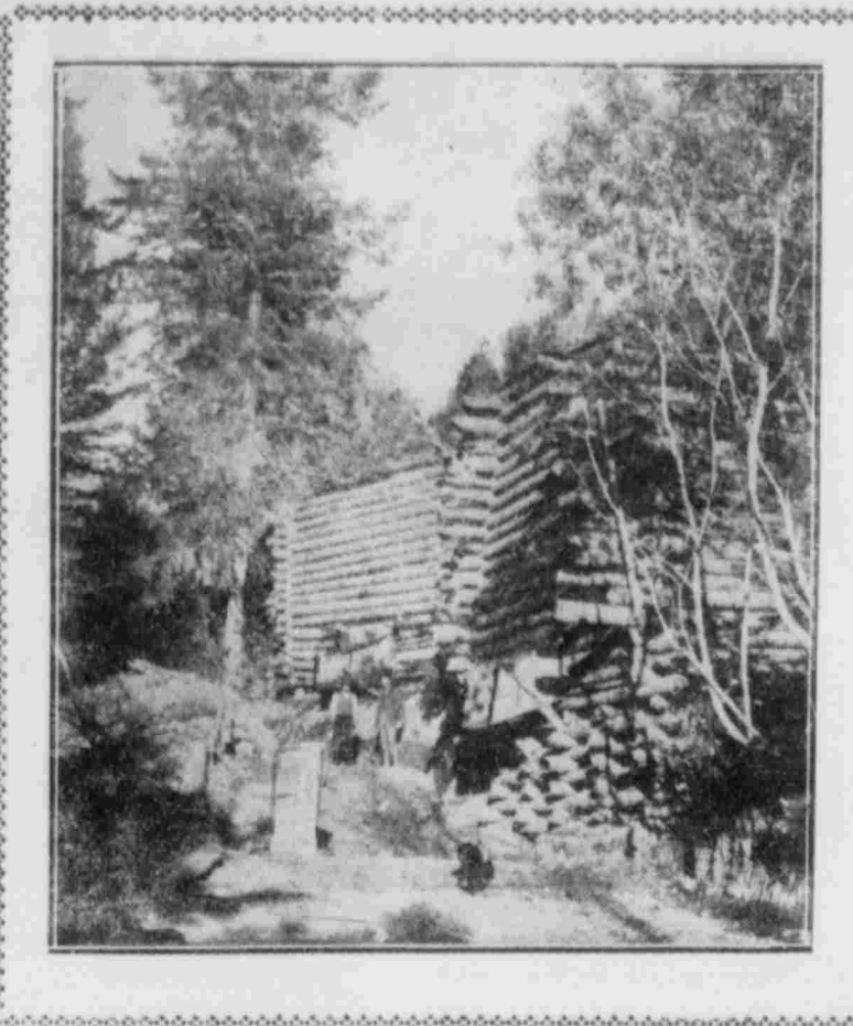
LOADING BINS, BROWN BEAR COAL CO.
