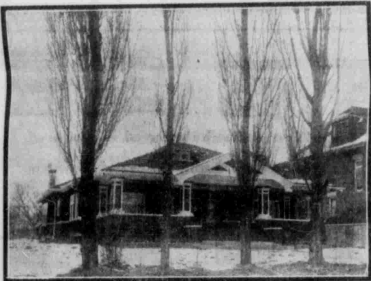
CLAUDE W. FREED'S BUNGALOW, YOUNG & SONS, ARCHITECTS.
