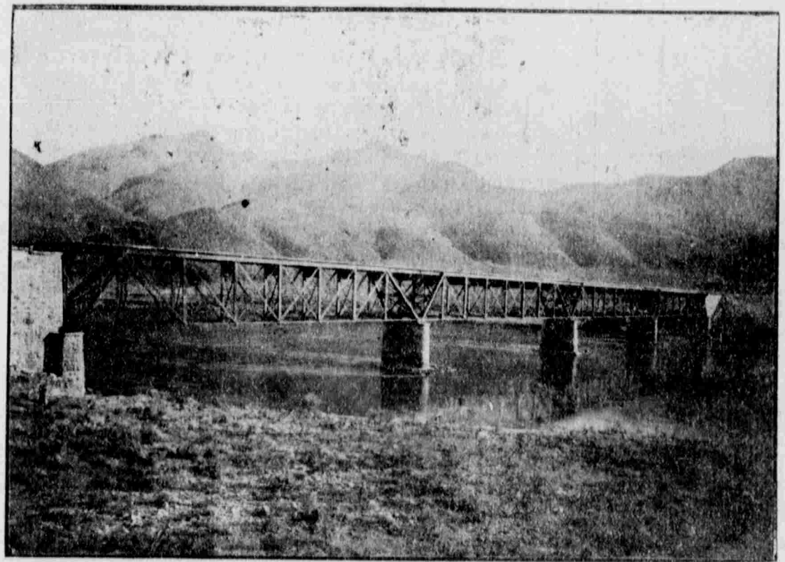
NEW OREGON SHORT LINE SNAKE RIVER BRIDGE.
