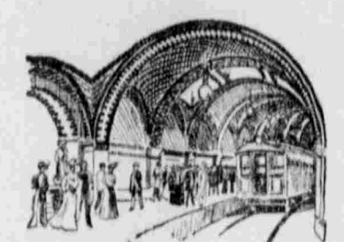
CITY HALL STATION, NEW YORK. Underground Rapid Transit.
