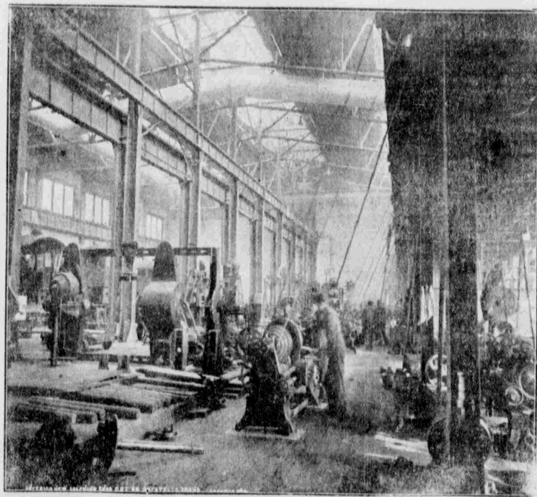
A CORNER OF THE MACHINE SHOPS.
