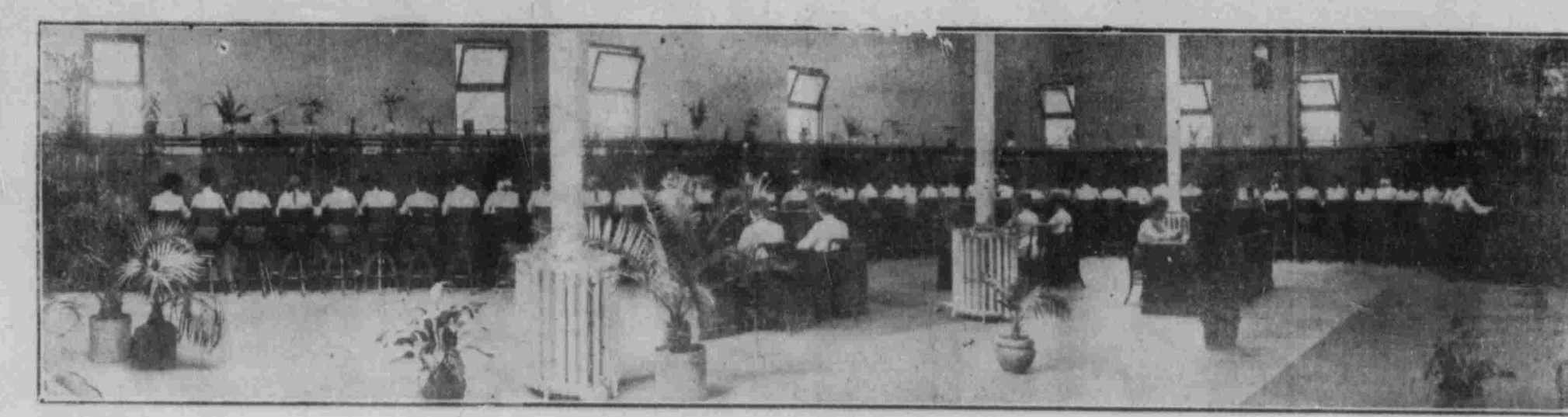
OPERATING ROOM OF UTAH INDEPENDENT TELEPHONE CO.
