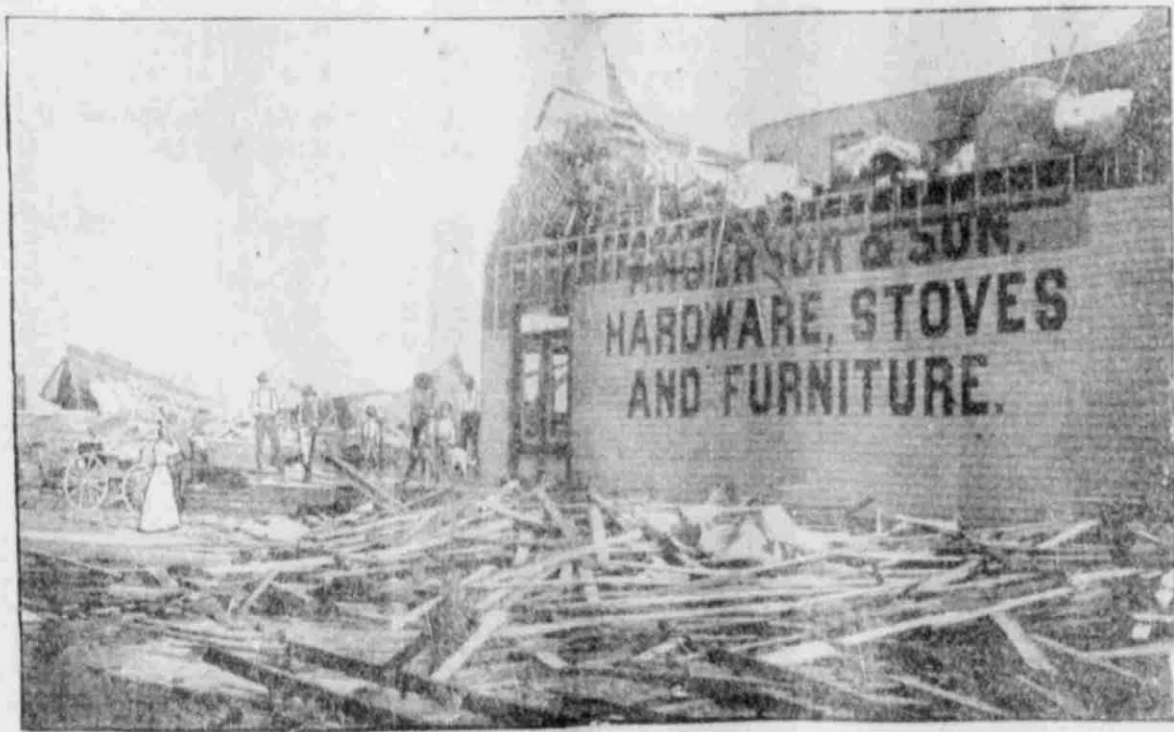
Here is one of the strangest freaks of the Galveston hurricanes. The furniture factory of Anderson & Son, Allyn, Texas, is unharmed so far as the lower story is concerned, but the entire top floor has been sliced off cleanly as if cut with a knife by the gale that slew so many thousands.
